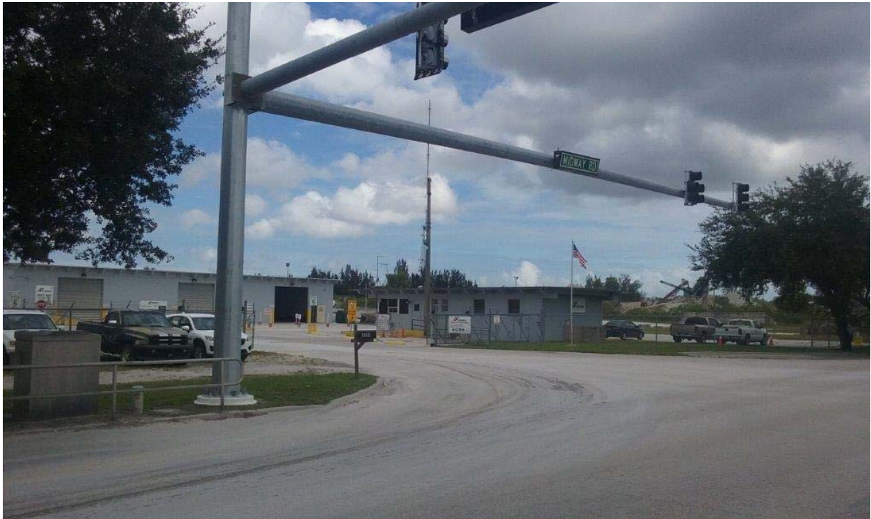
View to the northeast of entrance to Site No. 3 –CEMEX-West Ft. Pierce Ready-Mix & Block
