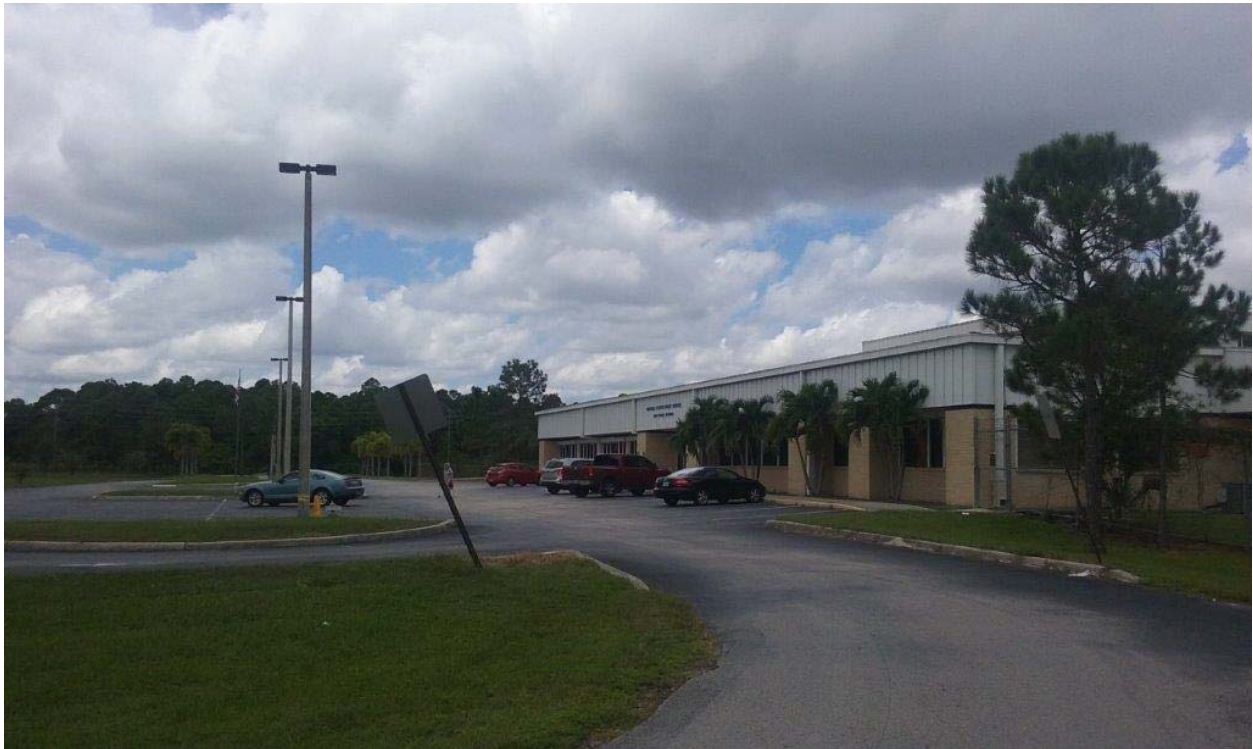
View to the northwest of Site No. 5 – US Postal Service
