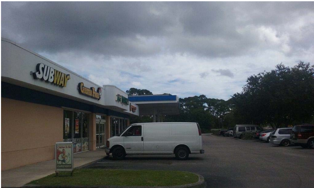
View to the west of Site No. 7 – Sunshine Food Mart #343
